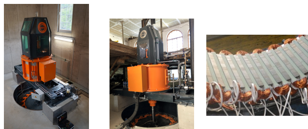
Fig. 2. Hydropower generator with corresponding coil winding
